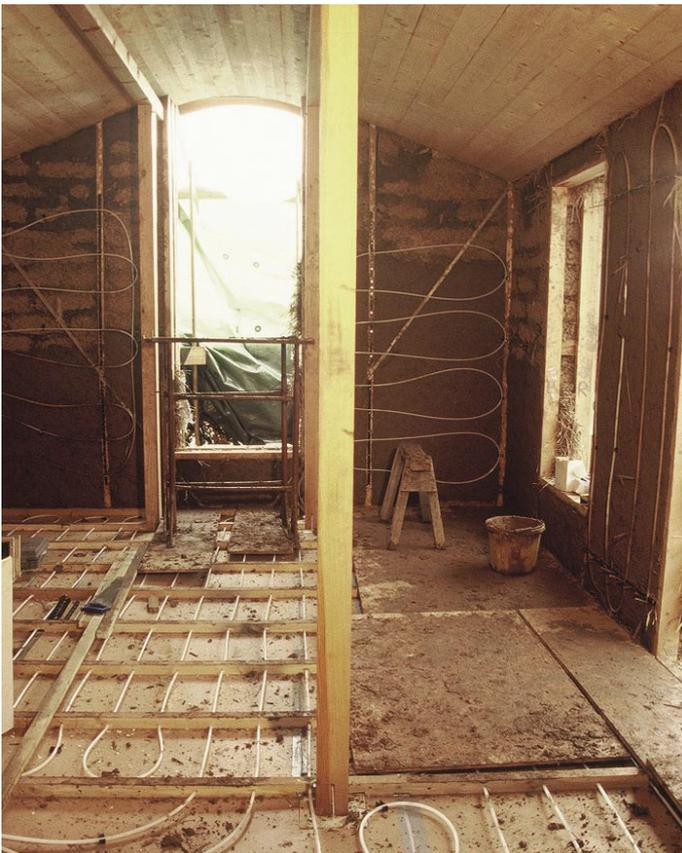
View of a Light Earth building incorporating heating pipes in the floor and walls. This creates a large surface of low level heating which has been monitored and proven successful in creating high levels of comfort. Design: Gaia Architects.
